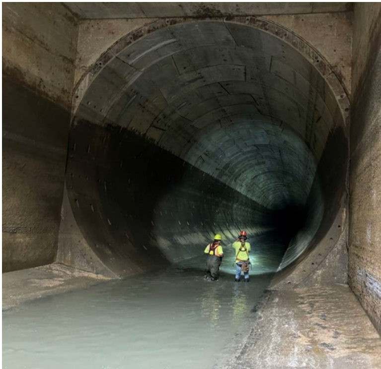
Figure 8 Ohio Canal Interceptor Tunnel (OCIT)
