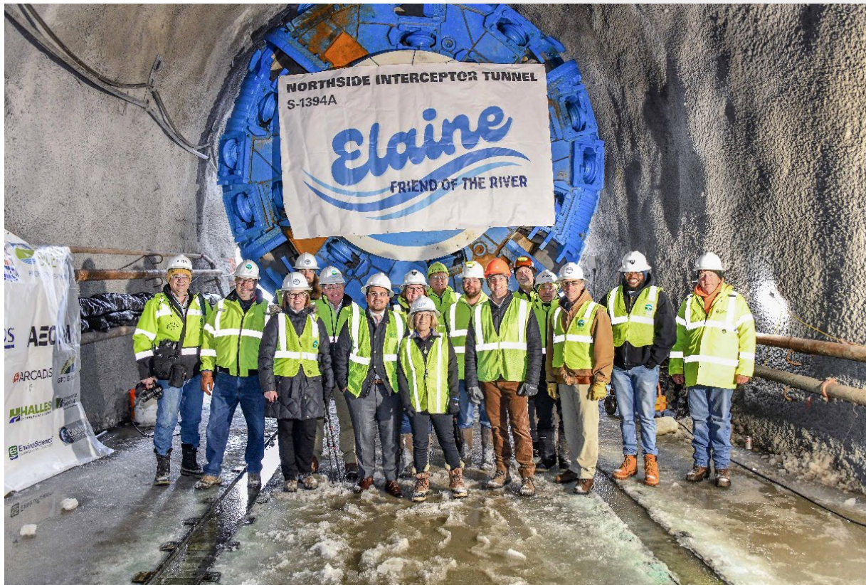
Figure 9. Northside Interceptor Tunnel Construction
