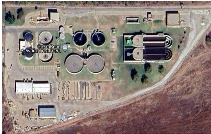
Figure 16: Great Bend WWTP
